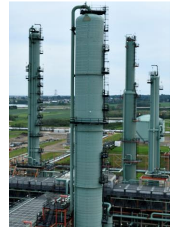
Condensate System & AEF
